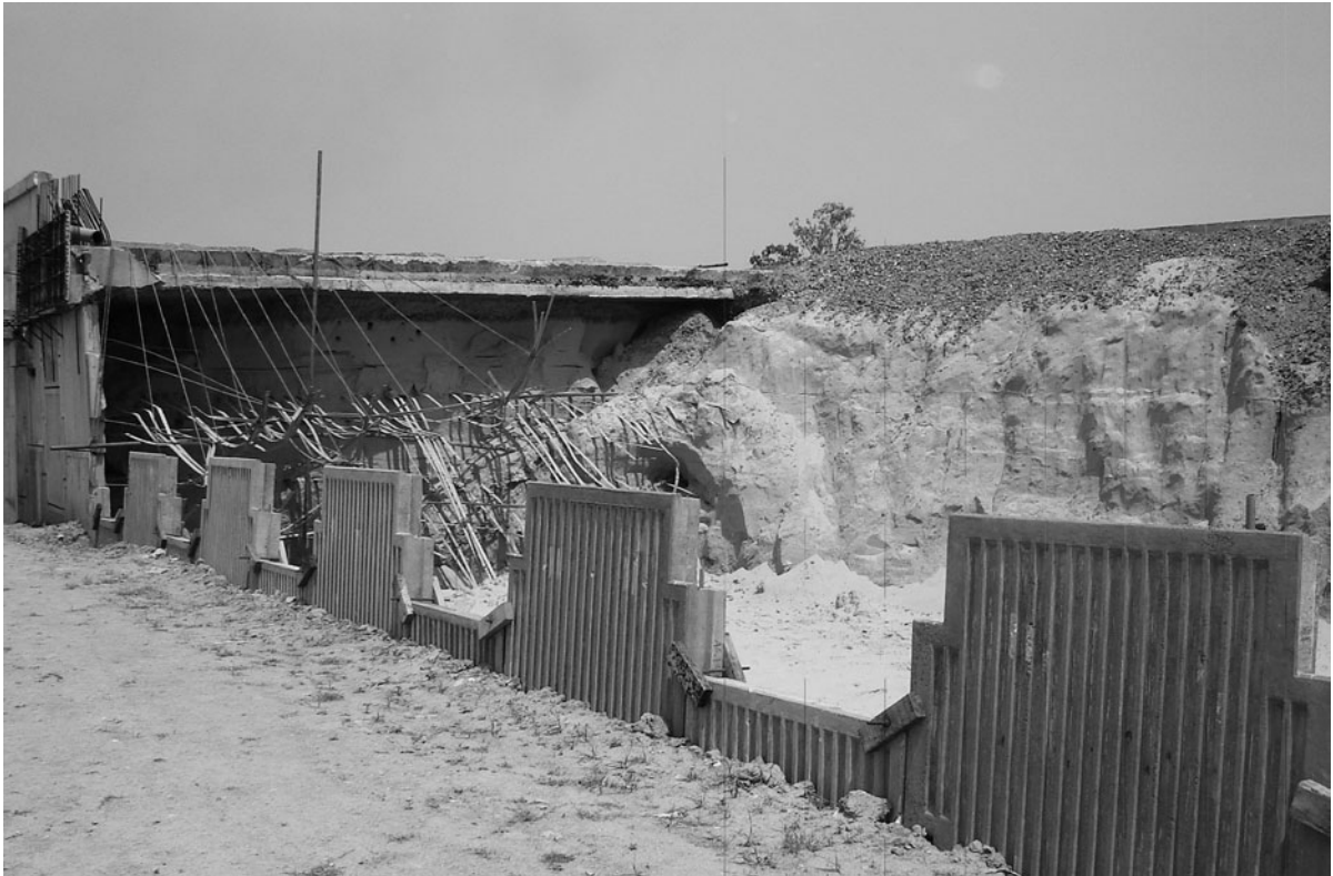
Fig. 1 Failure of the RE wall (note the exposed portion of the concrete bridge and the remains of the RE wall)
