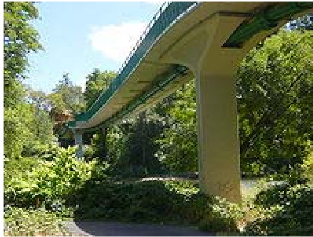
Stressed ribbon pedestrian bridge, Grants Pass , Oregon, USA
