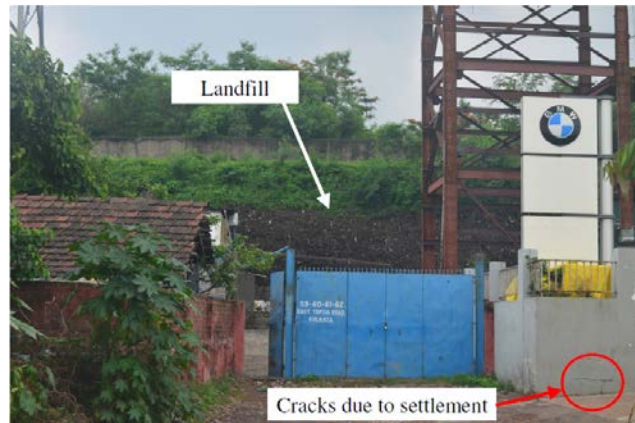
Figure 1. Facilities developed ca. 2011 over an inactive MSW landfill at Dhapa, Kolkata, India
